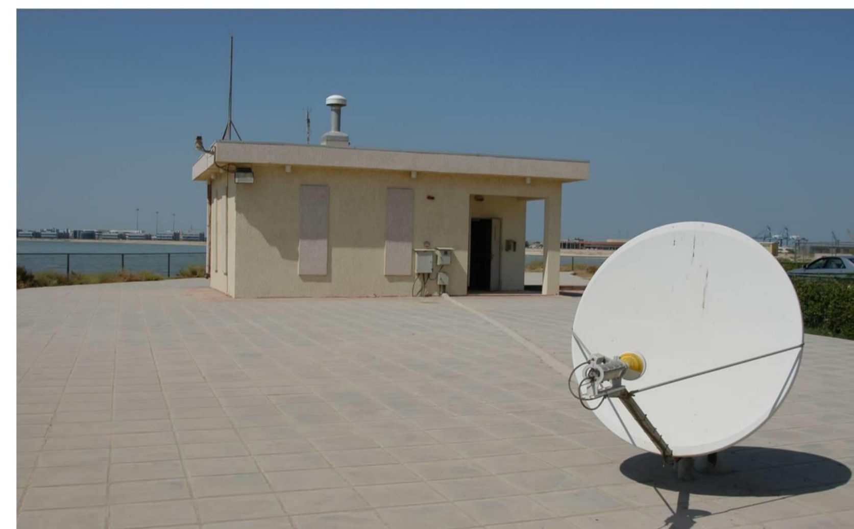
FIGURE 1: The building of station RN40 on the premises of KISR.
