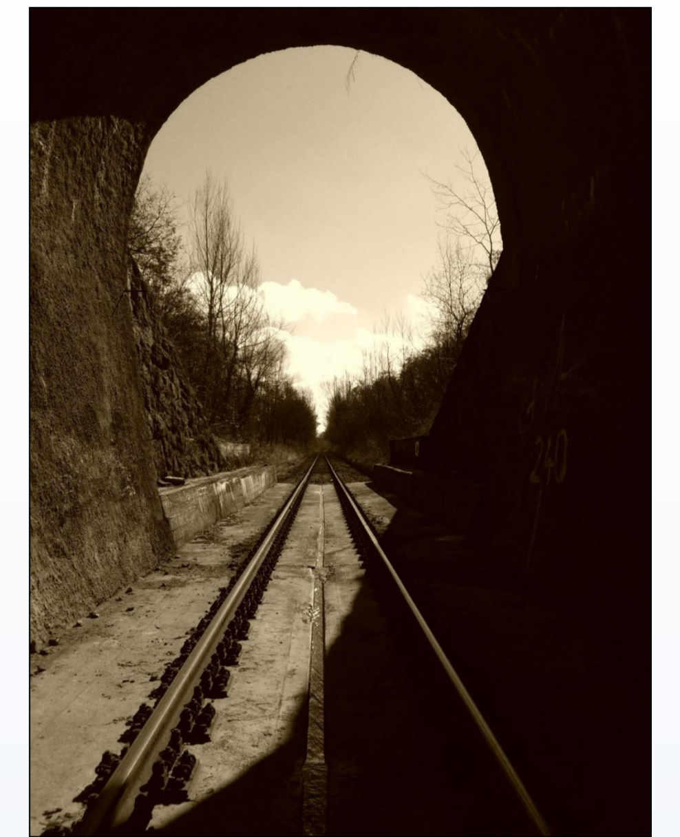
Figure 5. Southern tunnel arch
