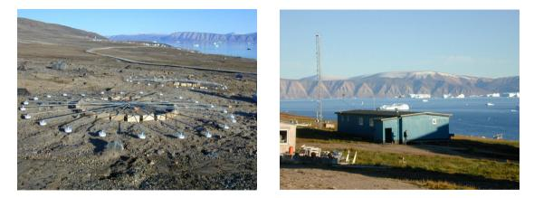
• I18DK is configured as an array of eight microbarometers allowing for direction CTBfrolest
