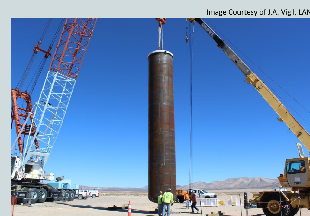
Emplacing a DAG chemical explosion canister (50 tons)
