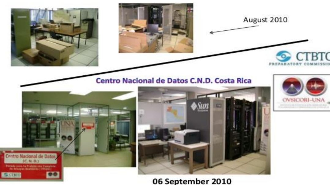
Figure 5. Installation of NDC-CR
