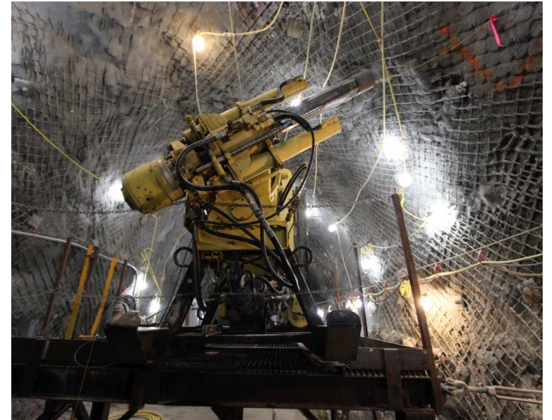
Borehole being drilled from adjacent tunnel to chimney for experiment's injection
